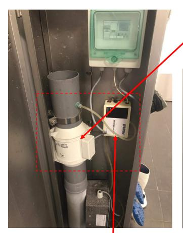
Elpress Ozone Generators connected to the Cylinder for odor control.
