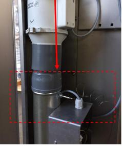
Controller – with Timing Switch. Refer to technical manual.
