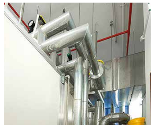
Chilled water ducting with green recycling ability.
