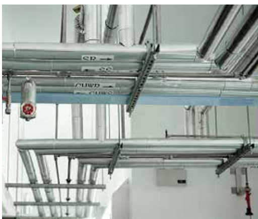
Chilled water (process) & steam distribution system.
