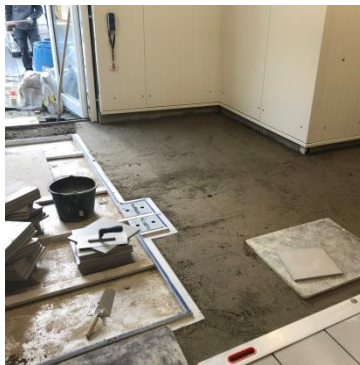
Sealing of drain
