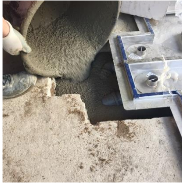
Sealing of drain
